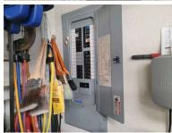
Service Entrance Type: Underground Panel Manufacturer: Cutler Hammer Location of Main Panel: Garage Main Panel Rating Amps: 200 Wire Types Found in Panels: copper
