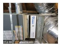
HVAC Filter Sizes: 20x25 HVAC Filter Width: 5 inch Filter Condition: Satisfactory
